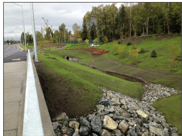
West Dowling Bioswale, looking west from Campbell Creek Bridge
