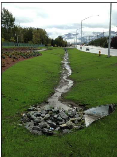
West Dowling Bioswale, looking east
